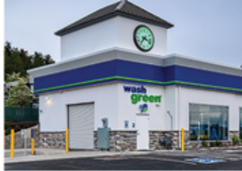
Car Wash Walls with Extrutech FORM Panels
